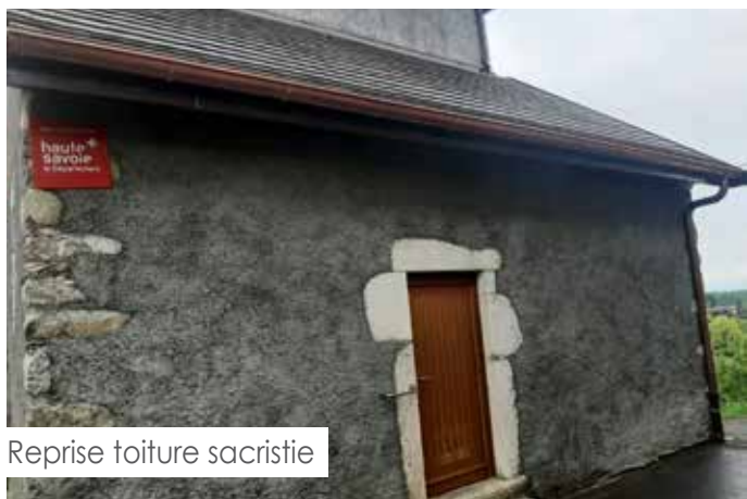
Installation filets pare-balls
